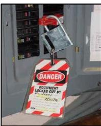
**Use Lock Out / Tag Out** program to ensure HVAC equipment cannot be operated during the spray foam process. For added safety, turn off all power.
