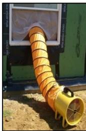
**Jobsite ventilation** is required during and for a period after the spray foam process. Keep the house under **positive pressure** (air needs to be coming IN to the house) to keep fumes out.
