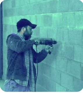
Using a 3/8" to 1/2" drive drill with a 3/8" or 7/16" masonry bit, begin drilling holes 4 courses off of the floor into the 3/8" mortar joint centering over the core of each half block. Holes should be drilled every 4 to 5 courses.
