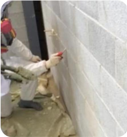
As the cores are filled, a tapered wooden dowel pin should be inserted into the fill hole once the tubing is removed to keep the foam from spilling out of the fill hole as the applicator moves down the wall.
